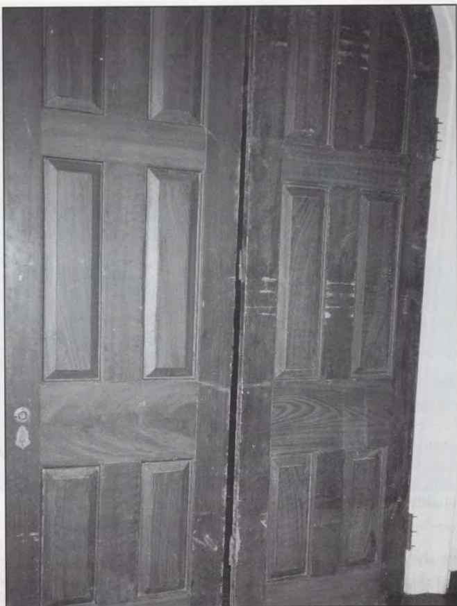
43. Detail of two sections of the double folding doors as they appeared when retrieved from their dusty storage place. The painted finish was obviously applied by a professional adept at achieving the appearance of the rich color and graining of mahogany. Rock Hall photograph.
