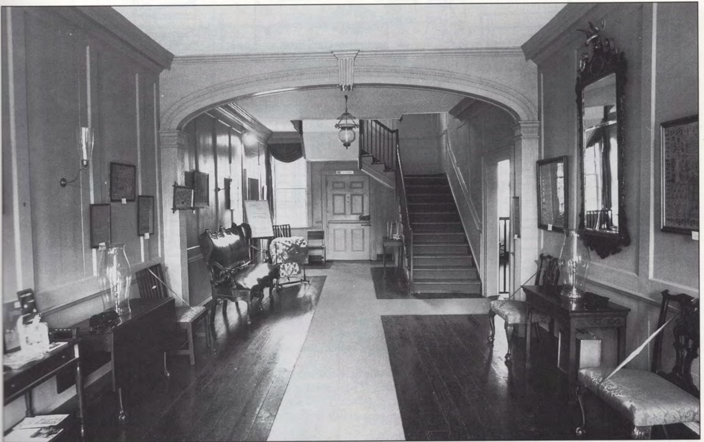
15. Top: View of the first-floor stairhall looking southward, showing the Federal-style archway and the new position of the stairs at the southwest corner. Photograph, SPLIA, 1976. Bottom: Details of the elliptical arch installed in the first decade of the nineteenth century. HABS drawing, 1935.
