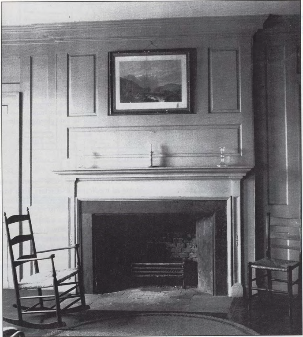
20. The southwest bedchamber had a new Federal-style mantel and flanking cupboard and closet storage areas installed. The room was given a fresh coat of white paint when this work was done in the first decade of the nineteenth century. The paneling above the mantel was left unchanged and has the distinction of being the only raised paneling in Rock Hall. Photograph, HABS, 1935.
