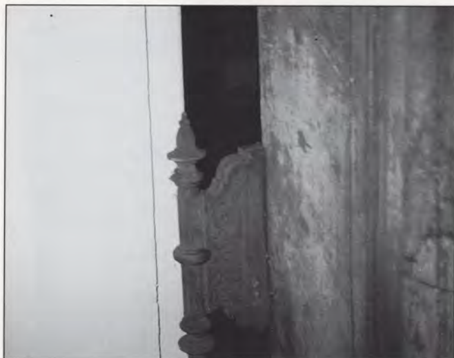
44. The distinctive ornamental heavy bronze butt hinges found on the long-lost doors were listed and illustrated in the 1871 catalog of the P & F Corbin Co. of New Britain, Connecticut. With bronze tips, as at Rock Hall, they sold for $13.50 a pair; with gilt tips they were $15.00 a pair. The mortise knob lock, which was designed specifically for use with folding doors, is of equally fine quality.
