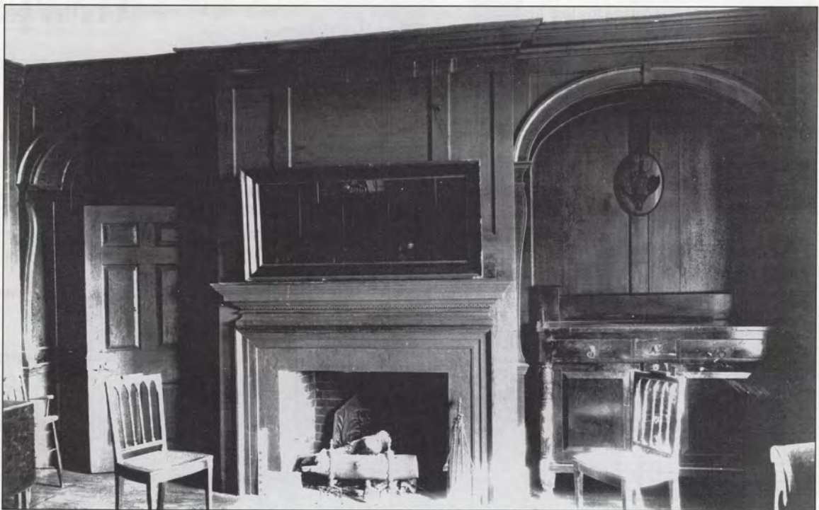
50. The mantel wall of the southeast parlor as it was altered in 1881 to replicate the southwest dining room. The door in the alcove at the left led to the east wing, where the new kitchen and pantry were located. Paint investigation indicated that it was the same door that was originally located between the east-side parlors and was displaced in this alteration by an archway. Photograph, HABS, 1935.
