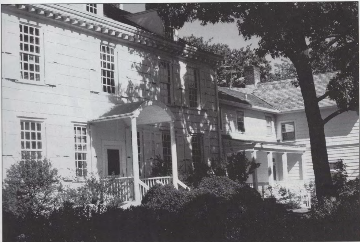
75. Top: This photograph captures the state of disrepair of the south porch at the time of the Hewlett gift to the Town of Hempstead. Photograph, Franklin Benkard, 1948. Bottom: The new south porch as designed by Otis Chapman. What materials could be salvaged from the old porch were reused, but a new design based on the north porch was followed. Photograph, Linda Barreira, 1993.
