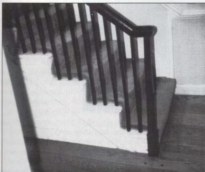
30. Architectural finishing details at St. George's Rectory, Hempstead (1793), are similar to those at Rock Hall that are part of the early-nineteenth-century alterations. Left: Simple square balusters and newel posts of the stair railing with blunt-ending handrails and half-newels attached to the stair wall beneath the chair rail. Top right: Decorative scrolls on step-ends. Bottom right: S-curved mantel fascia ornaments.
