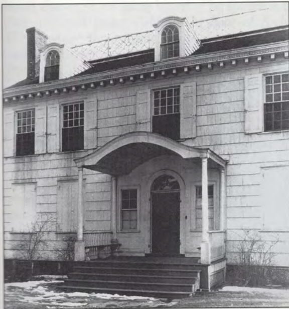
22. Photograph and measured drawing illustrating the similar roof forms of the new north porch and dormers. The round-headed windows with Gothic pointed muntins in the dormers appear in many of the pattern books used by builders. The type appears at Rock Hall well before similar dormer windows were installed at St. George's parsonage, Hempstead, the Platt-Lamb house at Fort Salonga, and the Joseph Lloyd manor house, Lloyd Harbor. Photograph and drawing, HABS, 1935.
