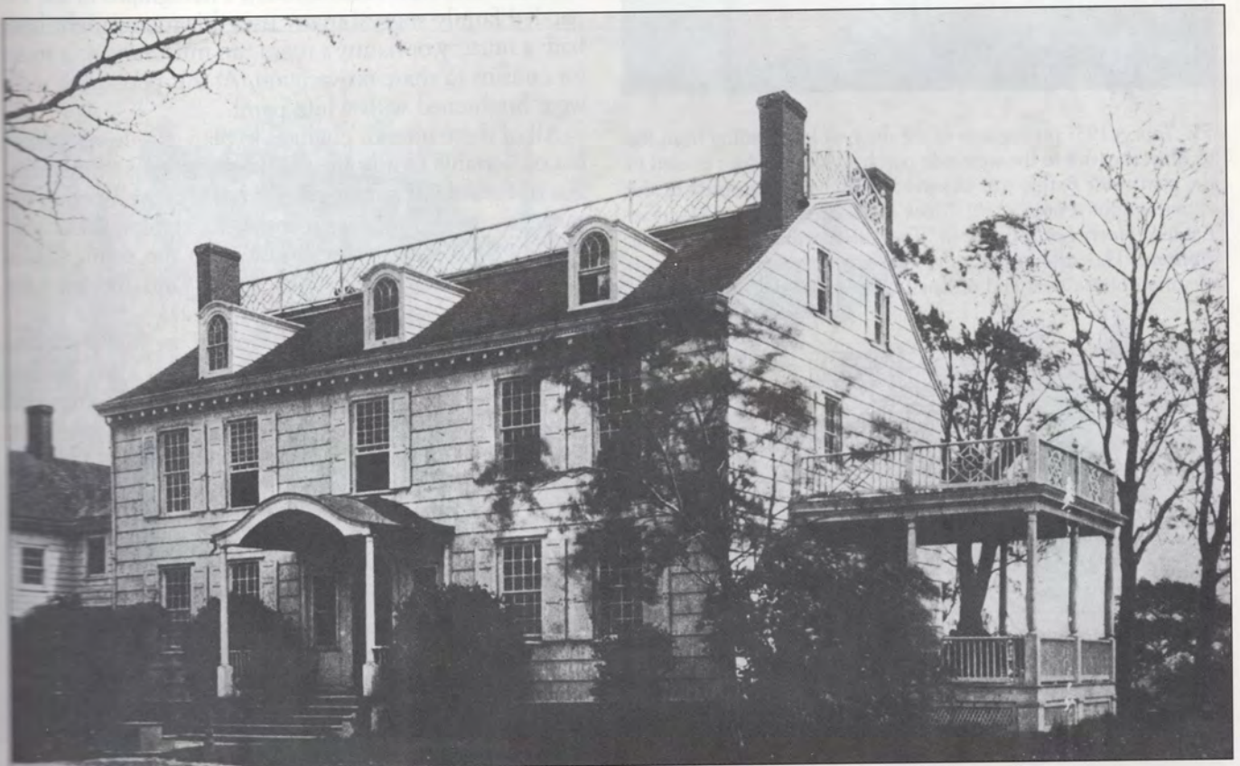
52. Rock Hall seen from the northwest. The new west-side porch was added in 1881 after the removal of the old slave quarters and deteriorated kitchen facilities. Doors with upper glass panels led to each of the west-side parlors. The unknown designer adapted and simplified the upper roof balustrade's "Chinese" design in a sympathetic manner on the porch roof railing.
